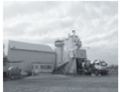
Ready-mix batch plant
